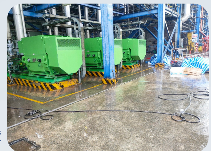
Installation & Alignment motor
