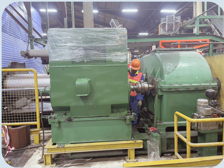
Installation & Test run DC Motor
