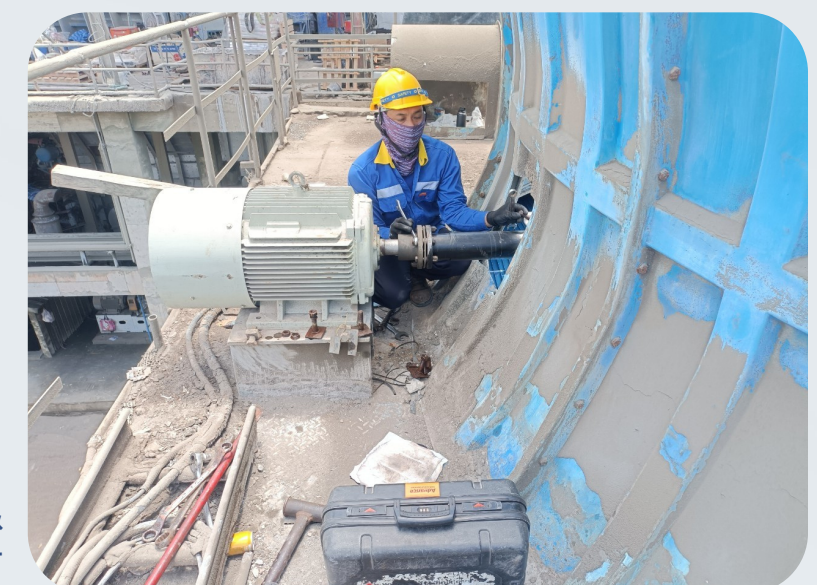
Installation Cooling tower & Alignment motor
