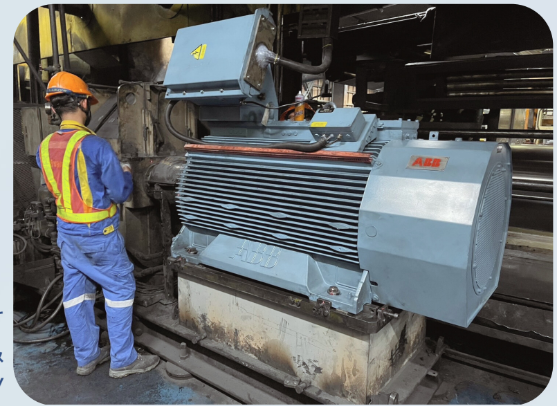
Overhaul motor Disassembly & Assembly
