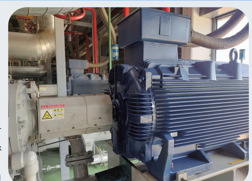
Installation Motor Compressor & Alignment Test run
