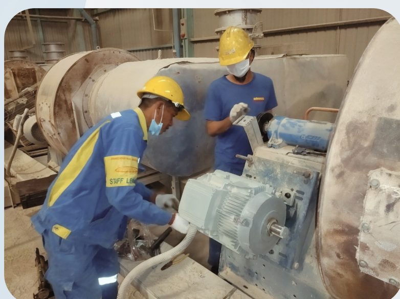
Dismantlement Installation and alignment
