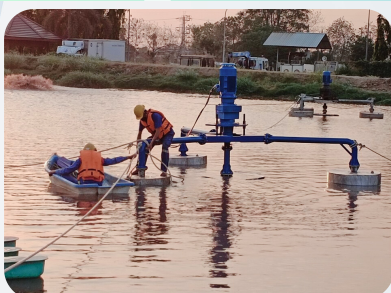
Installation Motor Aerator & Test run
